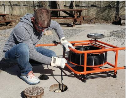
We're using the Flexi-Rooter more than our conventional cable machines. It handles most drain cleaning troubles – from root problems to grease and sludge stoppages.
