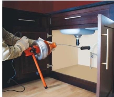
6. Repeat rocking the machine forward and back as you feed the cable into the line.
